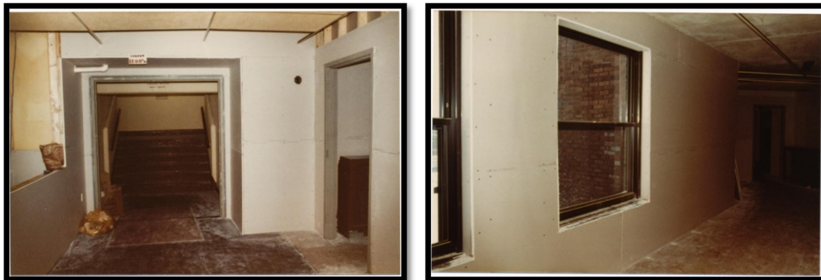
Duluth Bethel Building undergoing renovation, ca. 1970s
